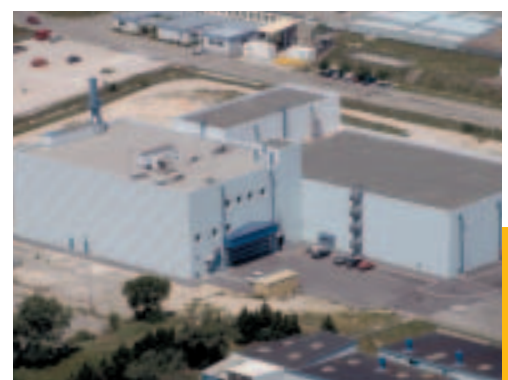
View of the multi-purpose storage facility (COGEMA Marcoule)
