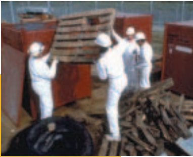
Decommissioning the Brennilis power plant
