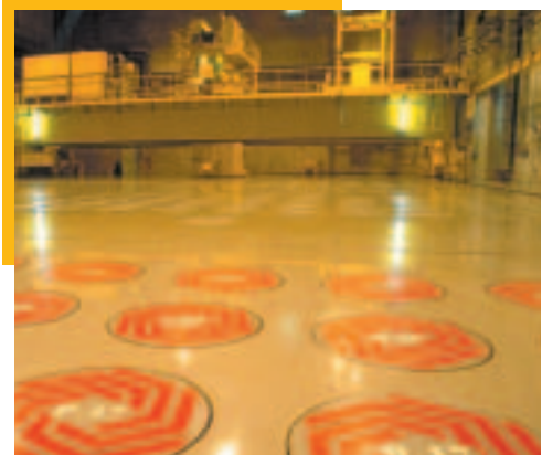
R7 - UP2-800 vitrification plant storage hall (COGEMA La Hague)
