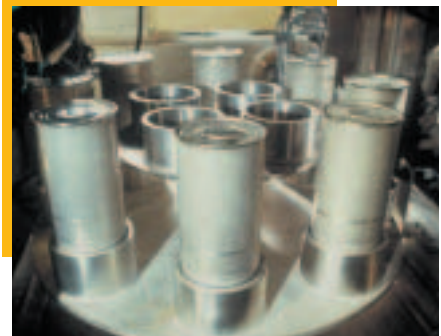
Carousel of plutonium boxes Mox Melox fuel manufacturing plant COGEMA Bagnols-sur-Cèze
