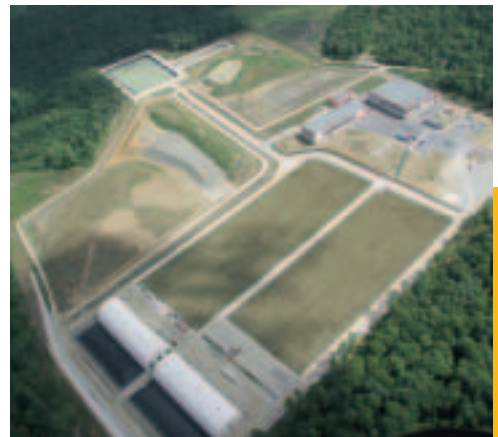
The Aube VLLW disposal facility
