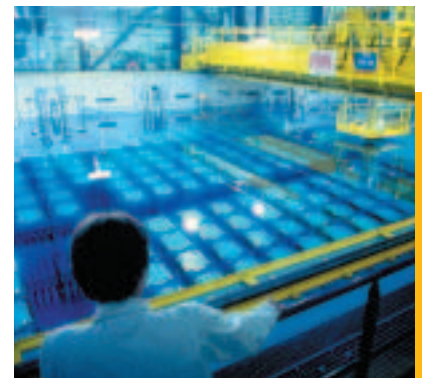
Spent fuel storage pool. Spent fuel reprocessing plant COGEMA La Hague
