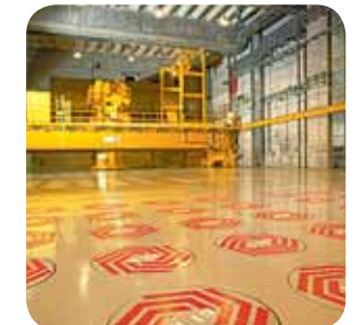
Storage of HLW in ventilated shafts on the AREVA site at La Hague, in the Manche
