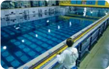
Before recycling, spent fuel is stored, in pools which facilitate its cooling
