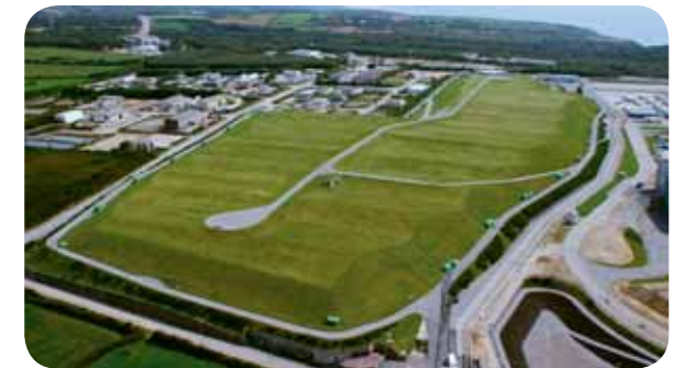
The CSFMA took over from the Manche waste disposal facility (CSM). It was the first French disposal facility and, from 1969 to 1994, accepted 527,225 m 3 of waste. Today this facility is closed and is subject to regular monitoring
