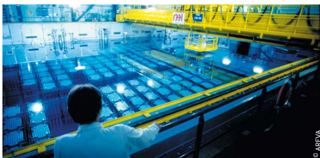
Storage of spent fuel in fuel cooling pool
