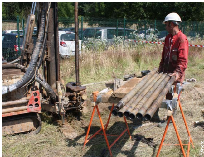
Borehole for geological investigations in view of finding a disposal site for LLW-LL
